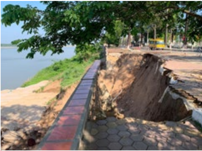
Fig. 43–46: Living with water in Kratié: The city's close relationship with its water resources and flood prone character are represented in the local architecture and riverbank erosion is a constant threat to infrastructure
